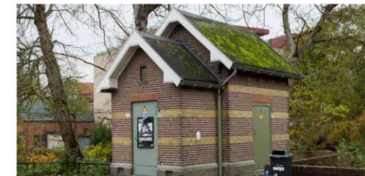
MS-MS station (3-23kV)
